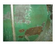
In this photo (left) the internal lining (green) is peeling off the inside of this UST and the tank walls are rusting.
